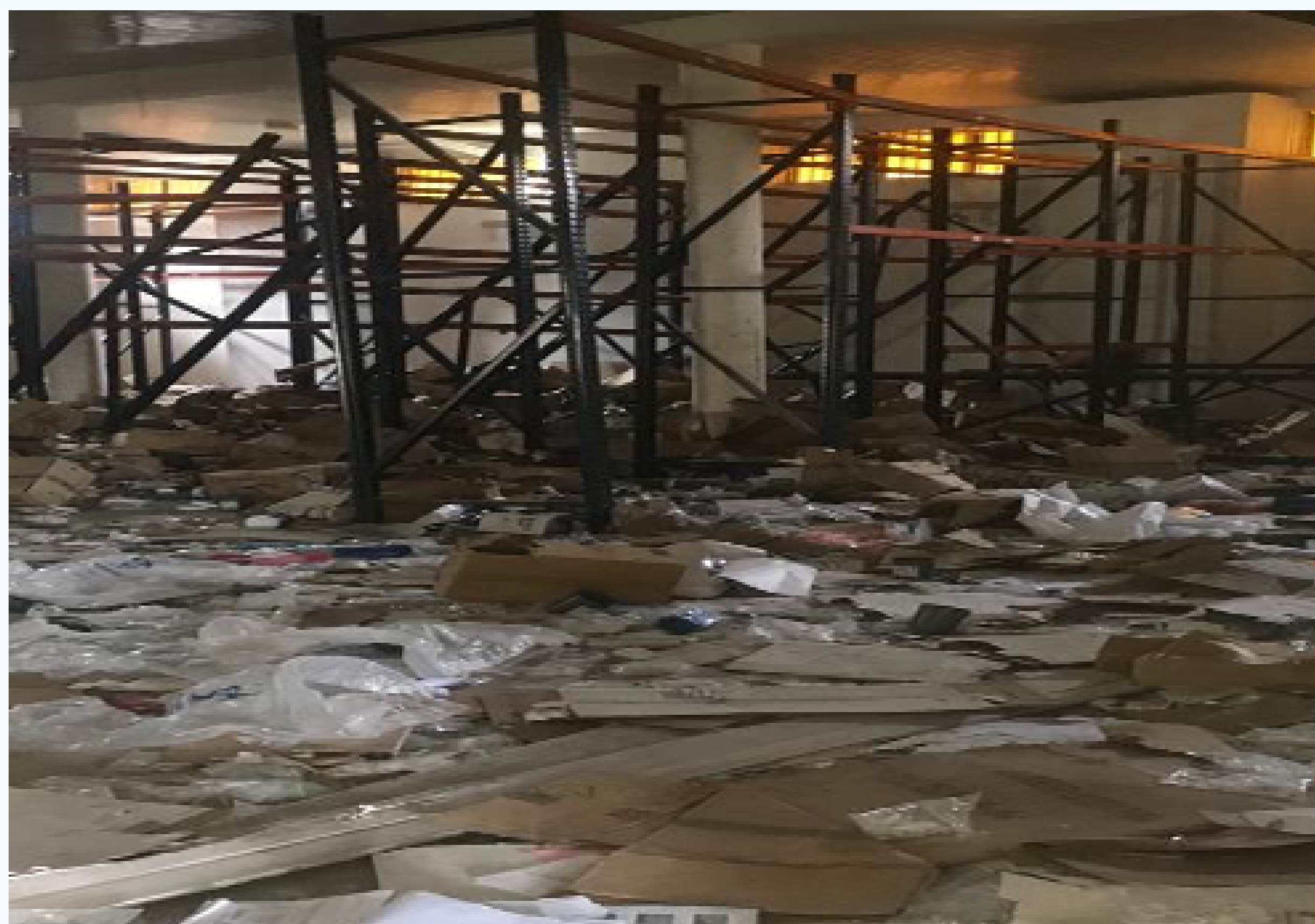
The Calabar axial warehouse after being vandalized.
